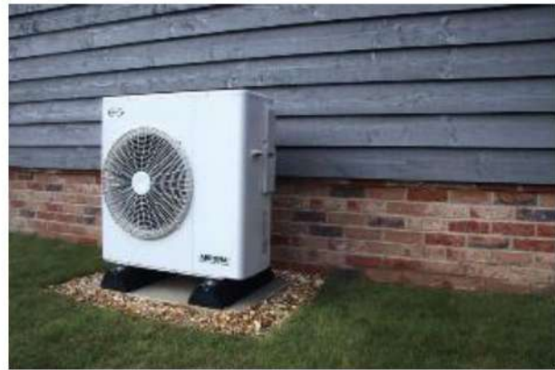
FIGURE 2: EXAMPLE OF A DOMESTIC SIZED AIR SOURCE HEAT PUMP
